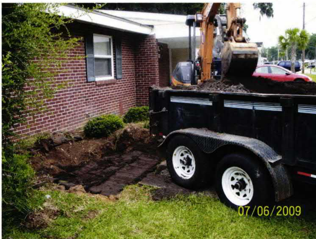
Picture 2: UST 1347 Cardinal excavation during backfill.
